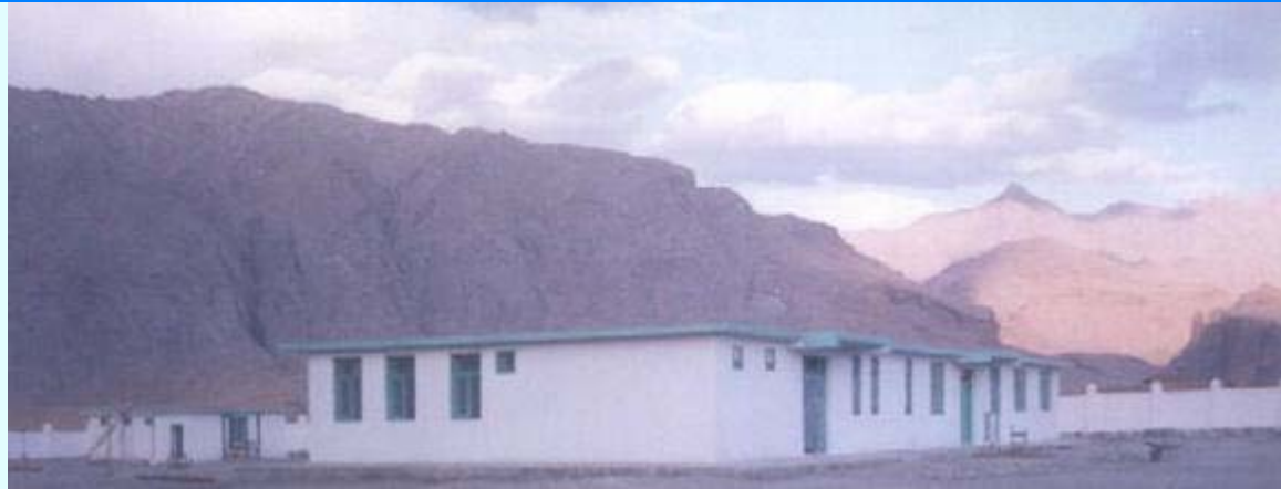
Gezab CHC newly constructed according to MoPH design
